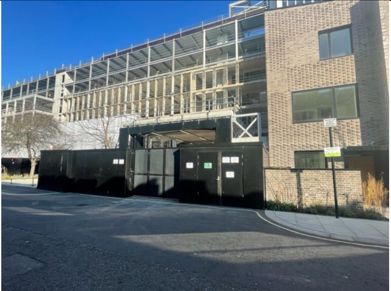
Loading Bay for 50 Eastbourne Terrace (& 40 Eastbourne Terrace) under construction in Chilworth Mews.
