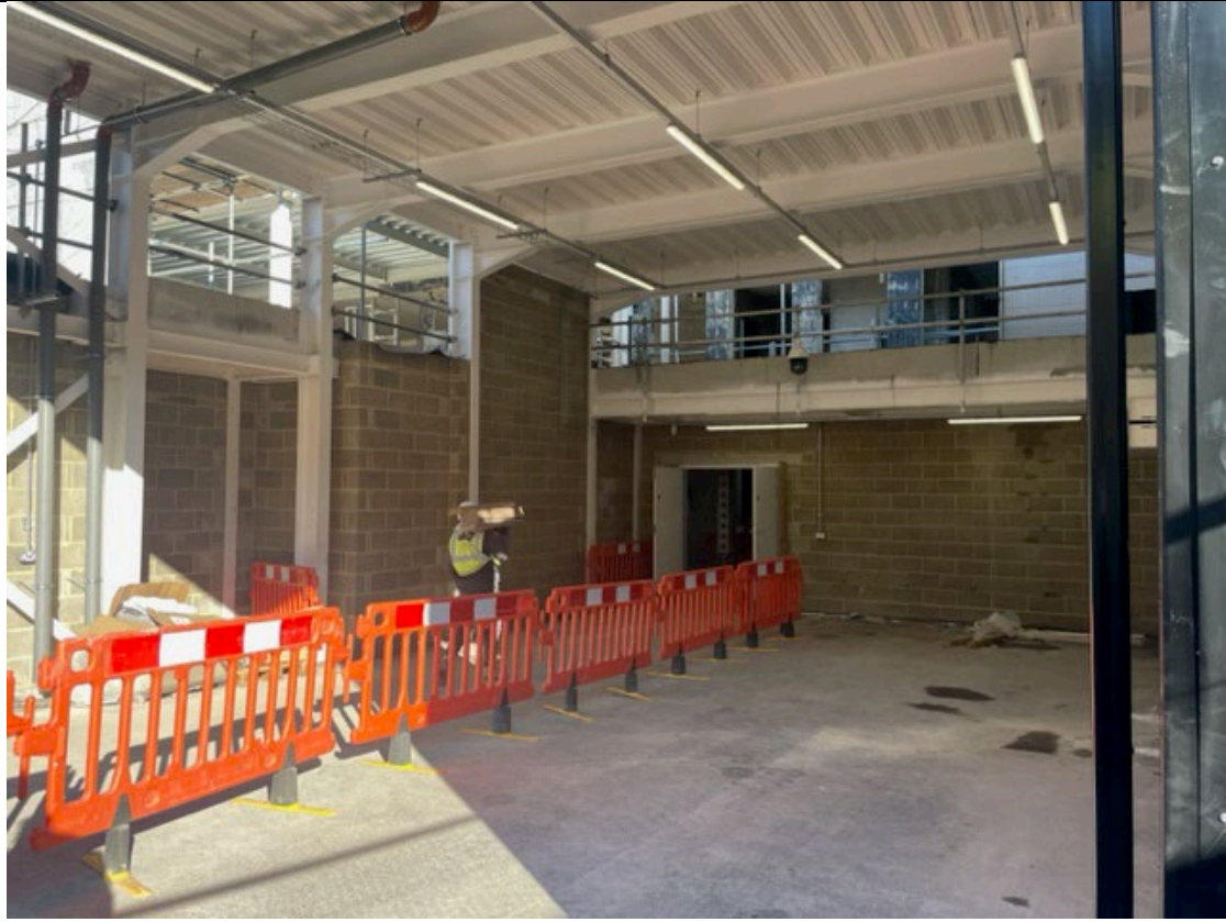
Internal area of loading bay
